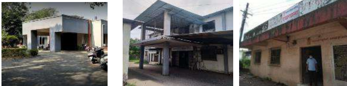
Figure 50 JNPA hospital, Jijamata Hospital and Raighad district polyclinic
