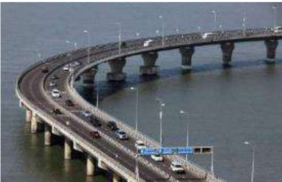
Mumbai Trans-harbor road link(MTHL)
