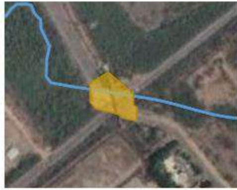
Structurally Weak Culvert
