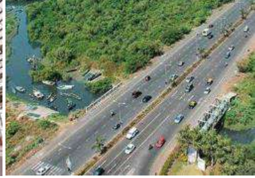
Navi Mumbai Coastal Road by CIDCO
