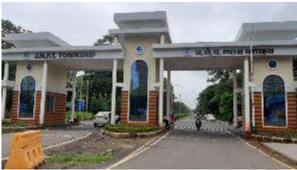
Main entry gate
