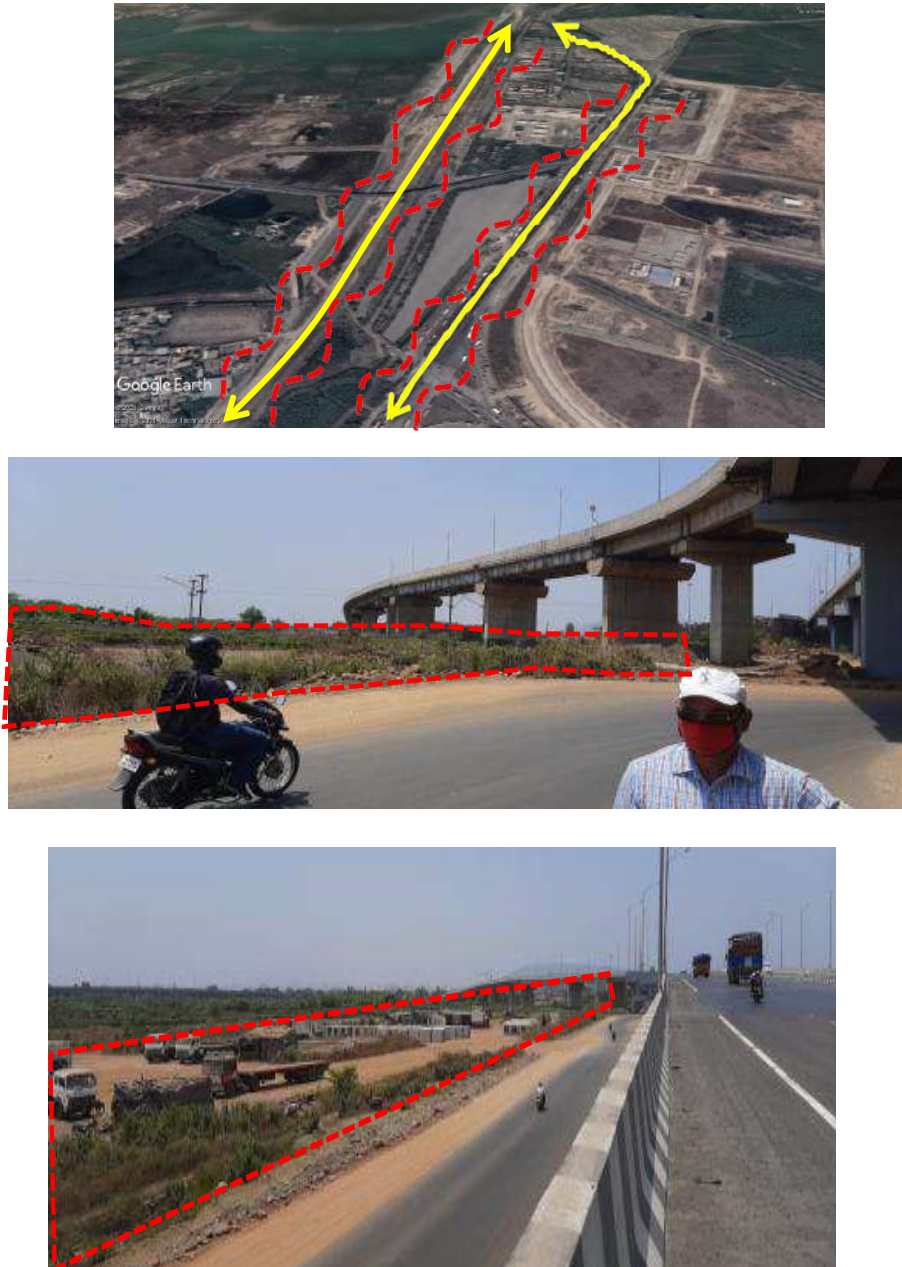
Figure 86 Photos showing road edge condition
