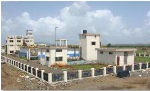
Figure 76 STP in SEZ area
