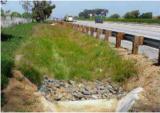
Figure 89 Diagram showing concept of Bio-swale
