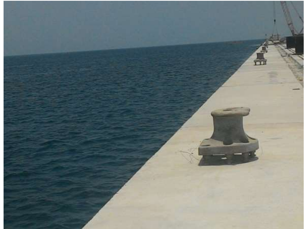
Bollards being installed at Phase 1
